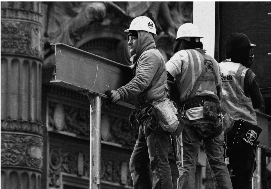
Construction workers in New York City in 2017 (Gordon Zheng/Wikimedia Commons)
